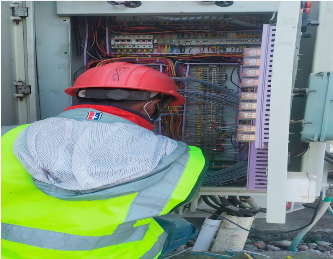
Figure : Working with safety ( Cumilla SS )
