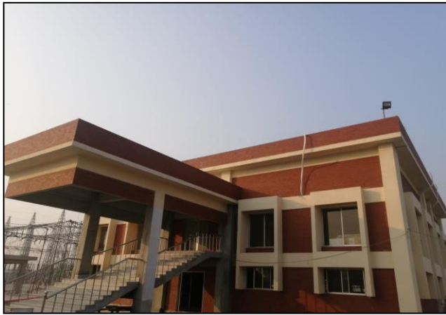
Fig-1: CRB of newly energized Kachua AIS ss
