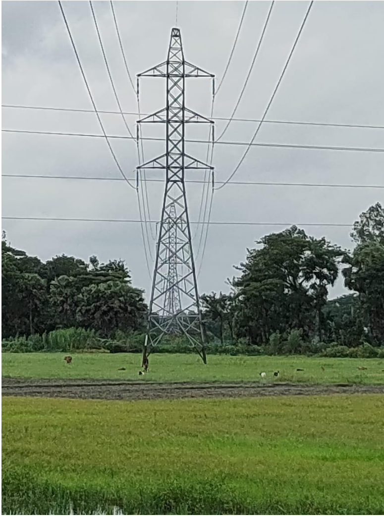
Figure: Site Reinstatement after rerouting of Cumilla-Chandpur Line
