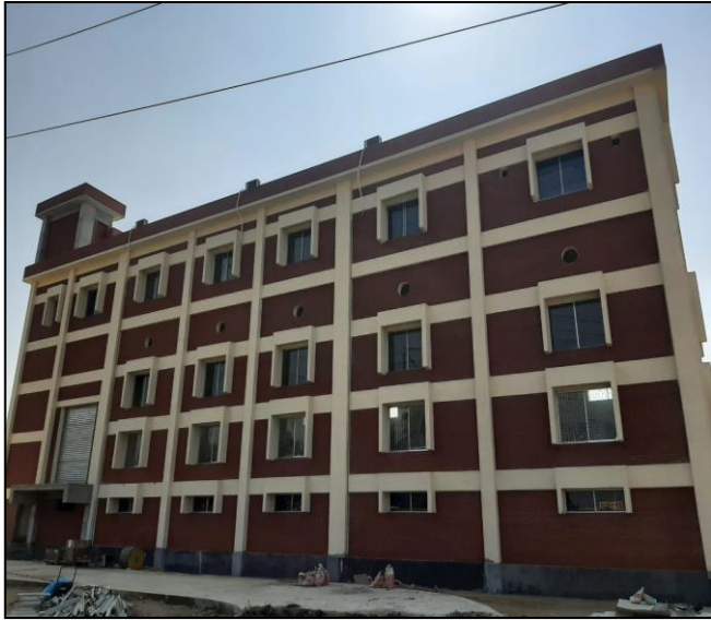
Fig-7: GIS building at Comilla(s) SS
